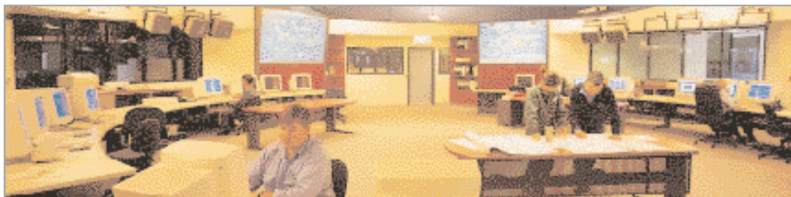
La sala controllo a Olympic Dam
